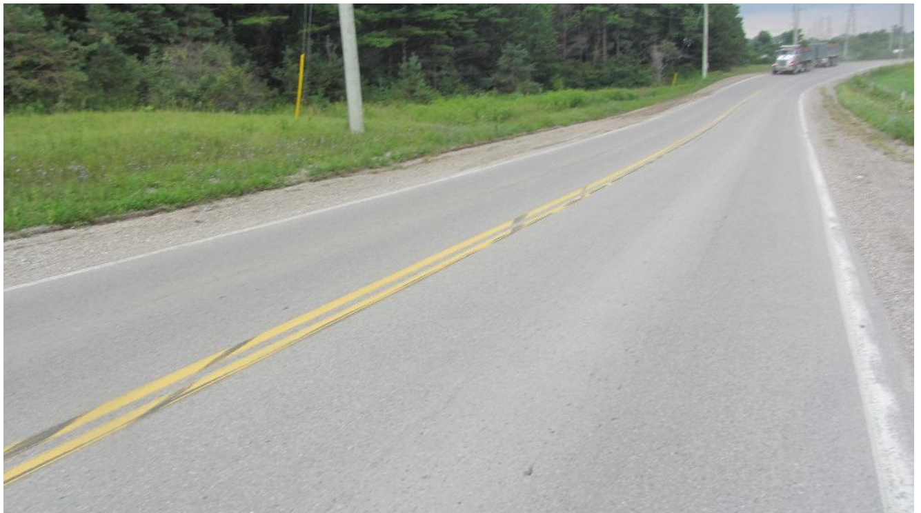
Figure 18: View, looking south-east, at the black yaw marks on the roadway centre-line.
