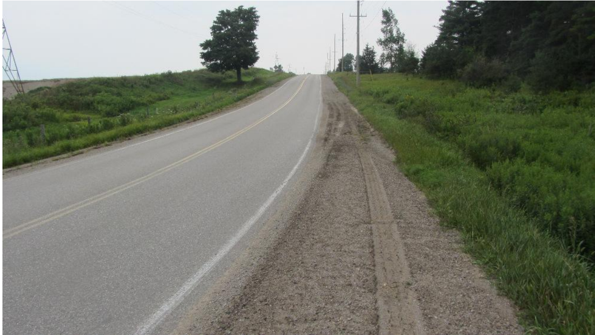
Figure 6: We already indicated that the northbound vehicle travelled onto the east shoulder so our first assignment is to detect where its tire marks are located on this east shoulder.
